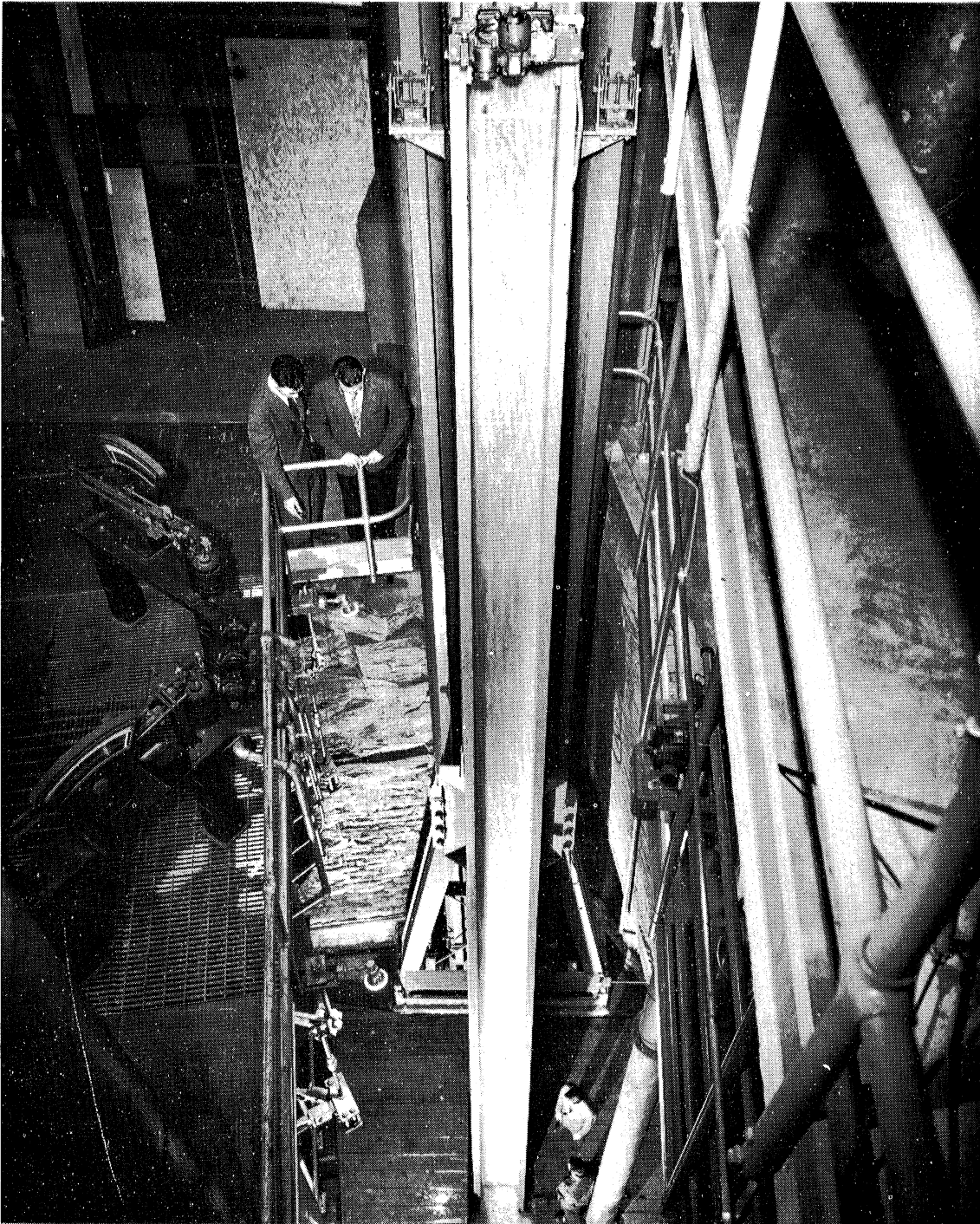
Fig. 3- Flume at 82\frac{1}{2}^{\circ} Slope Crosses Four Laboratory Floor Elevations Vantage Points for Photographic and Visual Observation Available Throughout Flume Length
